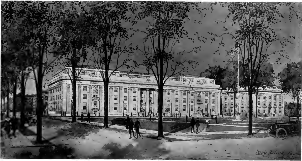
COMMUNITY BUILDING, FLINT, MICH. DAVIS, McGRATH & KIESLING, ARCHITECTS
